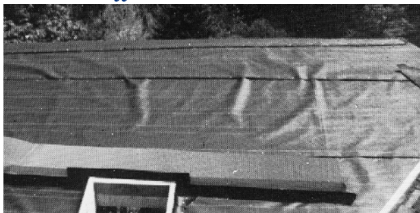
Conventional organic felts can telegraph wrinkles through the roof shingles.
